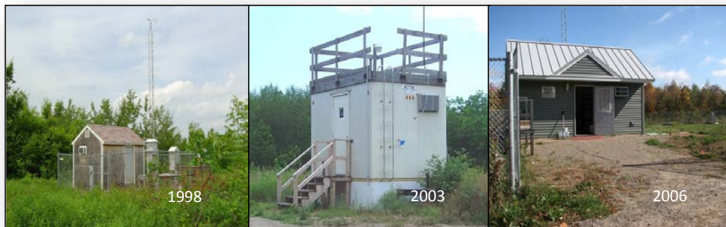
FCPC Air Monitoring Buildings
