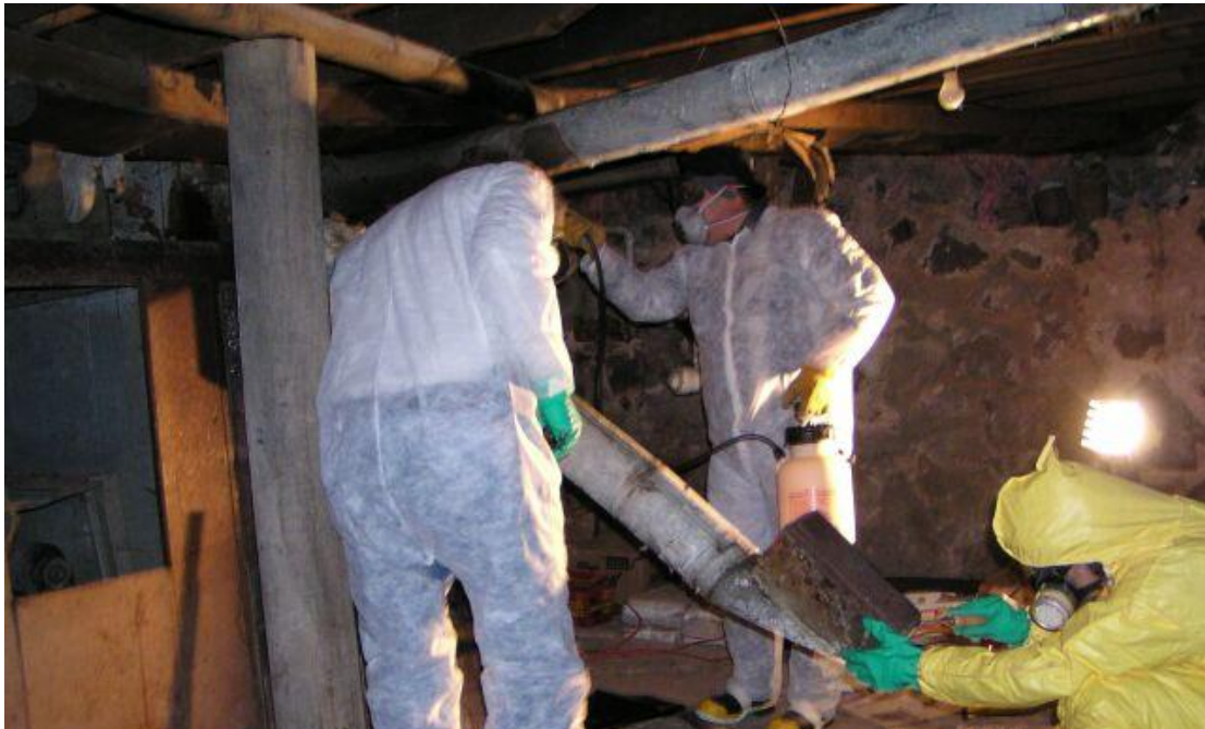
Pictured is the department director, a Tribal maintenance worker and one of our fire department personal, working to remove asbestos from the basement of an old Tribal building. They are shown fully wetting the material, then double bagging it for disposal at the county landfill.
